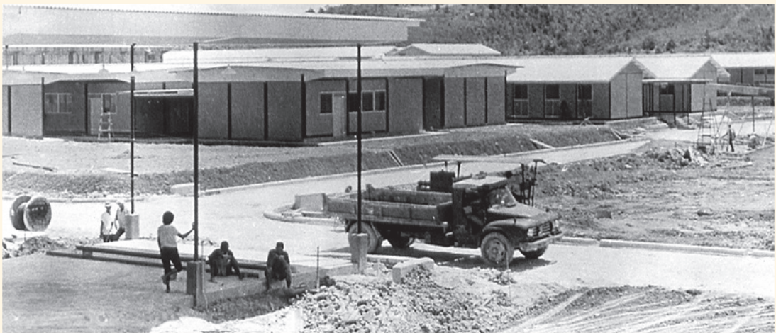
A view of the first Institute HQ buildings from the MT Lines.
