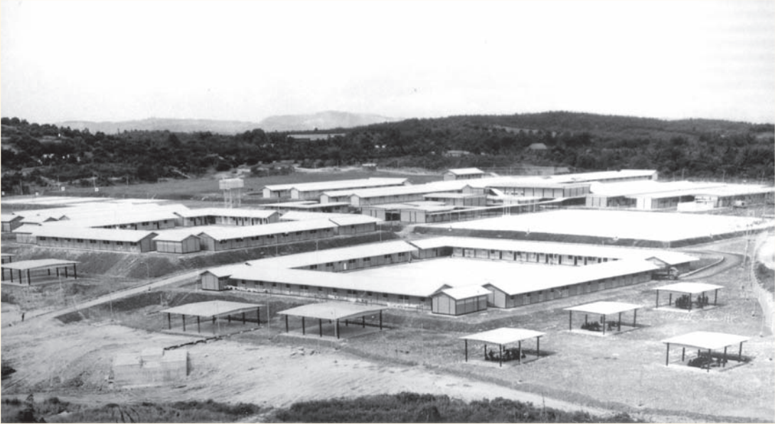
SAFTI buildings under construction near Pasir Laba junction in 1966.
