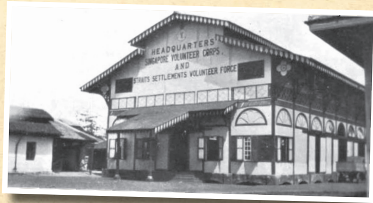
Drill Hall, SVC Beach Road.*
