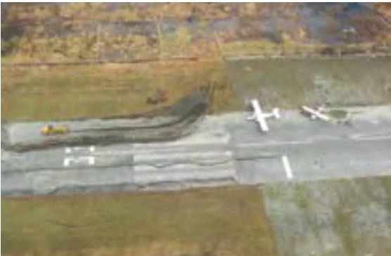
The earthquake cracked the runway at Meulaboh's only airstrip 16 km from the town. Only small airplanes and helicopters could use the 6,000-foot airstrip safely. Another hazard was the narrow road that led to town, which had collapsed in several places.
